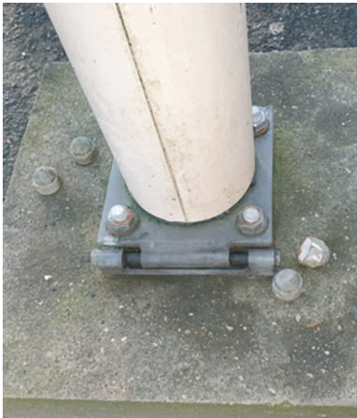
Check Anchor-plate Fittings
